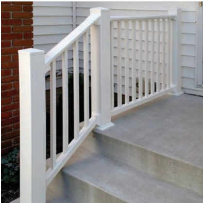
Standard Baluster 7/8" x 1-1/2" Rectangular Vinyl 2-7/8" Baluster Spacing
