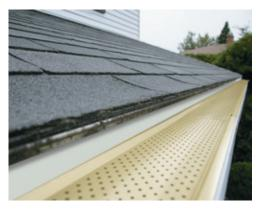
Over the years, the building industry has tried to solve the issue of hanging gutters. The solutions haven't been good ones. It started with spikes and ferrules, which can work loose and be bent by a fallen tree limb or heavy snow. Today's typical choice, hidden hangers create weak spots and gaps and leave flimsy gutters prone to warping and denting. Worst yet, the warping can lead to water infiltration and damage the roof, fascia and foundation.
